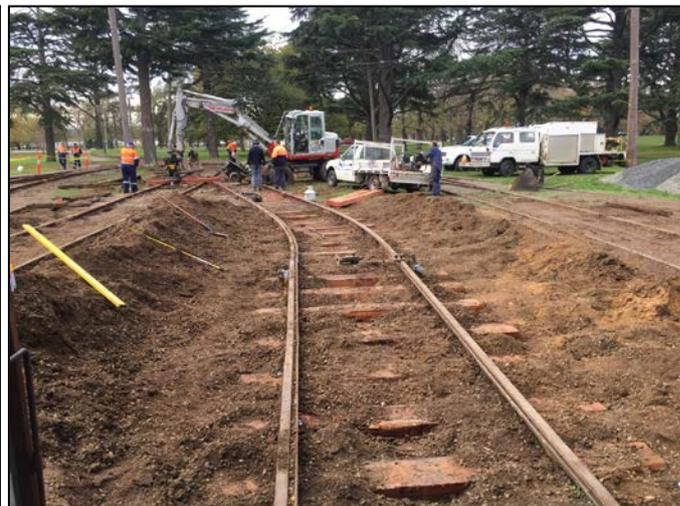
**Above:** Once the track had been dug out it was obvious that most of the original sleepers would need to be replaced. Already 100 new sleepers have been installed with 6 & 7 roads still to go.
